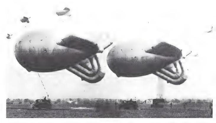
Barrage balloons being raised. They were anchored to the ground with steel cables, and often posed as much of a hazard to friendly aircraft as they did to enemy aircraft.
